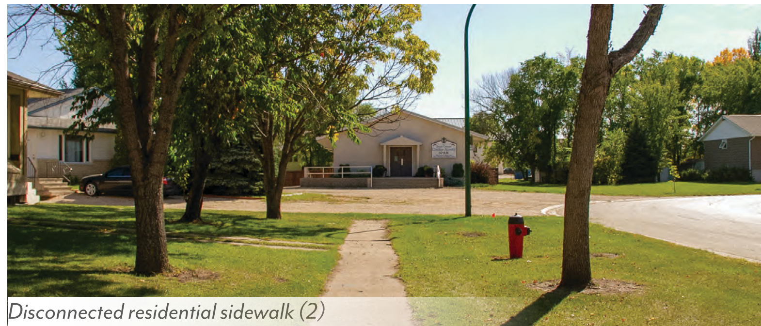
Disconnected residential sidewalk (2)
