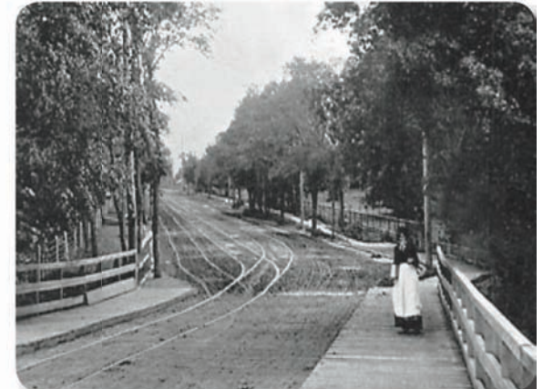
Osborne Bridge looking south, 1903. U of M Special Archives, Illustrated Souvenir of Winnipeg.
