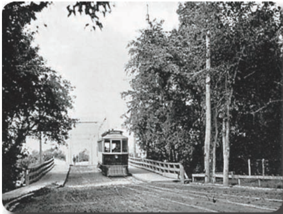
Osborne Bridge looking north, 1900. Heritage Winnipeg Special Collection.
