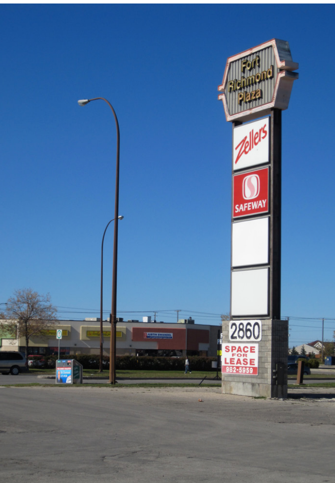
Present Fort Richmond Plaza
