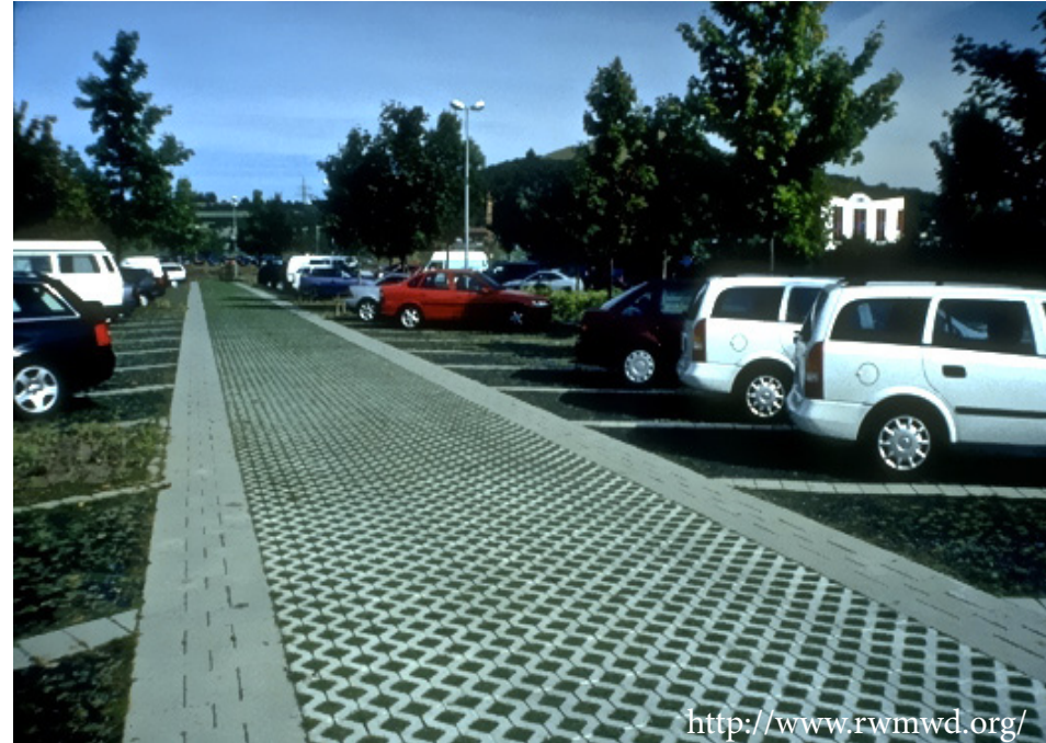
A green parking lot with povious pavement
