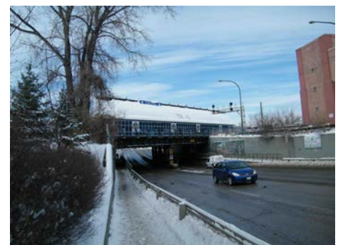
Underpass at North Osborne Street
