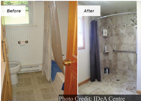
Figure 3: Modified roll-in shower with an installed grab bar
