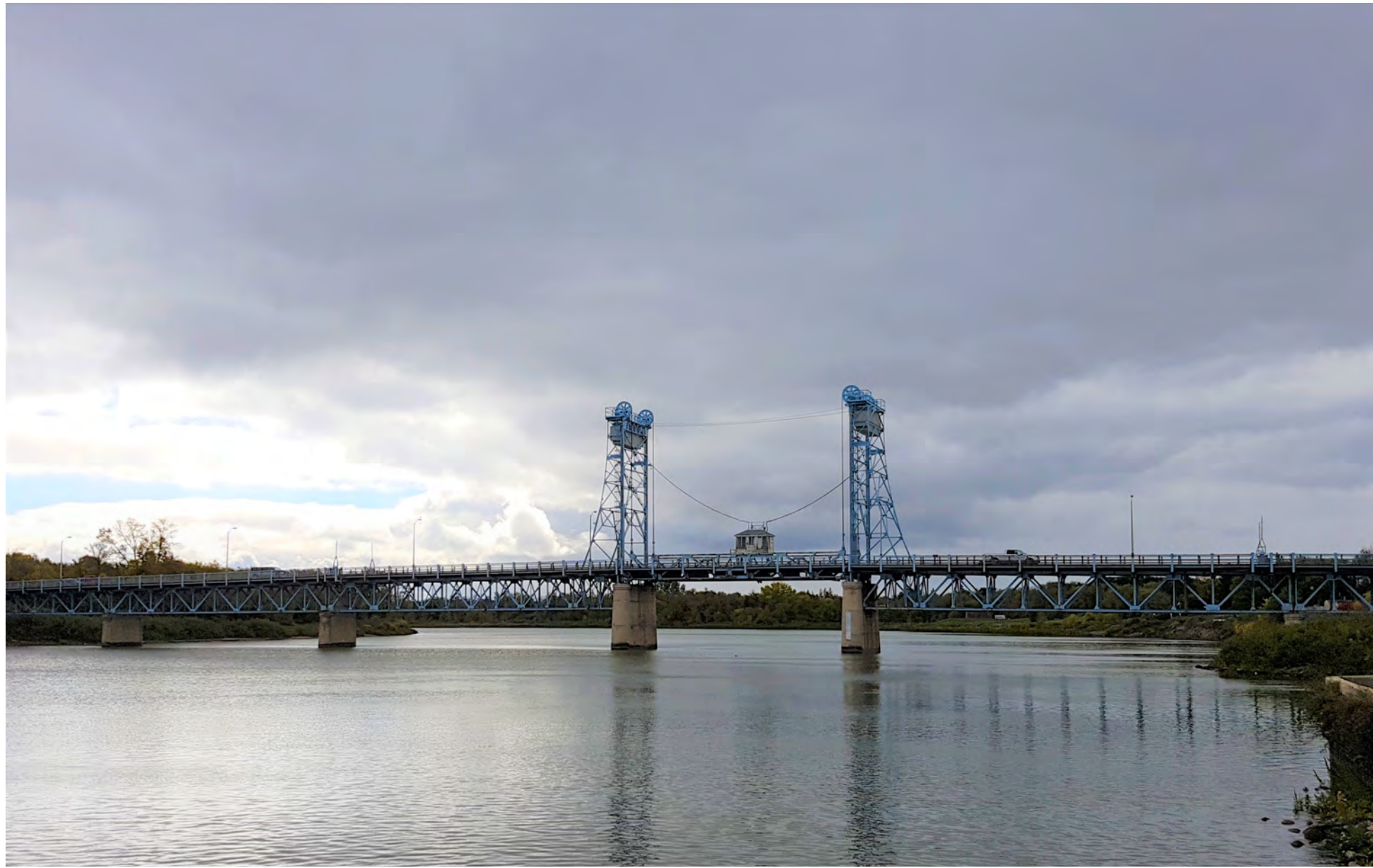
The Selkirk Lift Bridge is an iconic landmark unique to Selkirk and serves as a connector to rural communities and Winnipeg.
