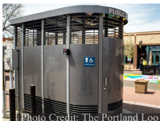
Figure 1: Portland Loo Unit
