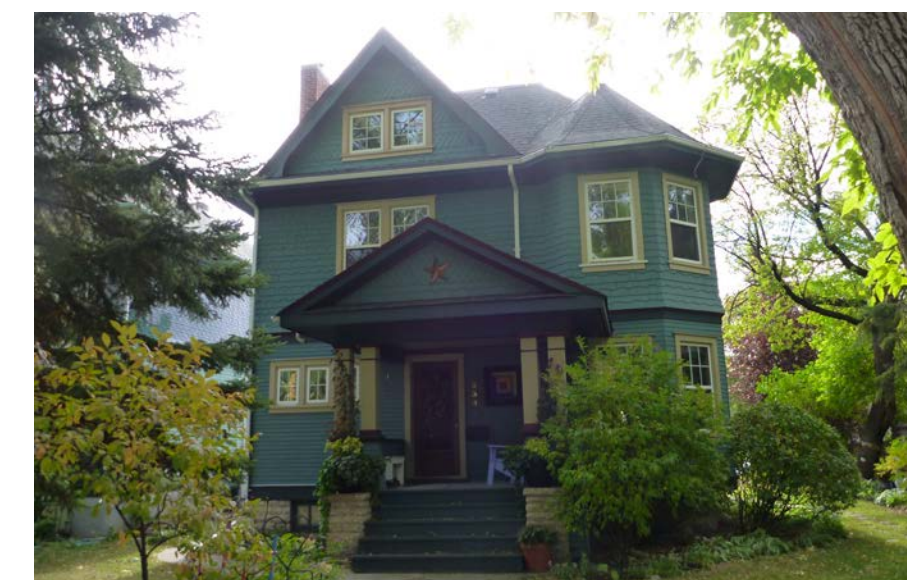
Some homes are maintenance heavy
