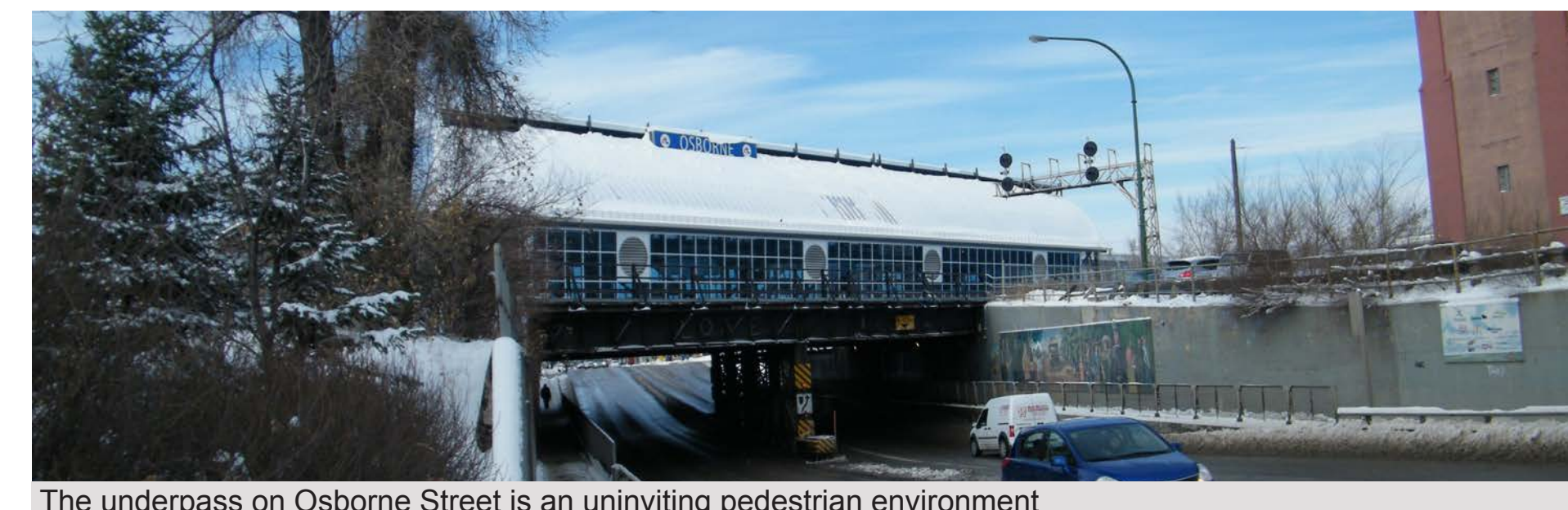
The underpass on Osborne Street is an uninviting pedestrian environment
