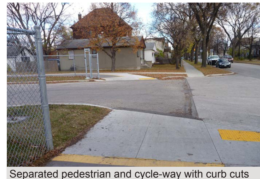
Separated pedestrian and cycle-way with curb cuts
