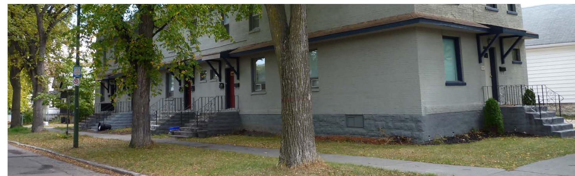
Steep stairs required to enter apartments are not age-friendly
