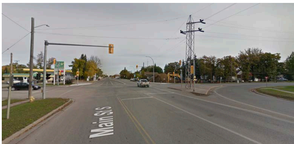
Figure: 45. Manitoba Hwy 16 and Manitoba Hwy 5 intersection in Neepawa, MB. (Google Maps)
