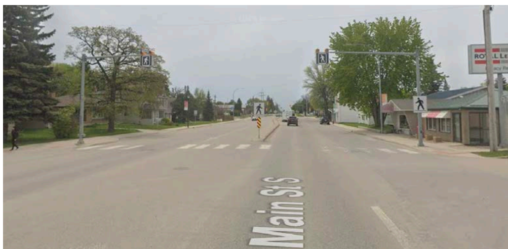
Figure: 46. Pedestrian corridor in Carman, Manitoba, across Manitoba Highway 13. (Google Maps)
