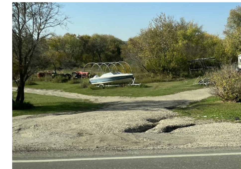
Fig. 33. Uneven sidewalk Photograph by Alandra Barairo
