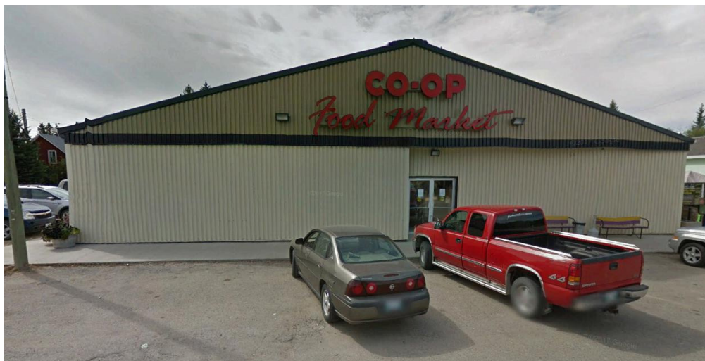
Figure 4-40. Example of a building mural - Sandy Lake Co-op
