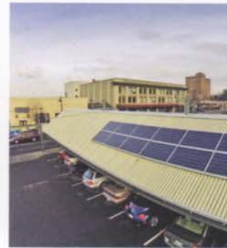
Figure 5: Shelters double as covered parking structures. (Photo Credit: Puget Sound Energy/Flickr, 2011)
