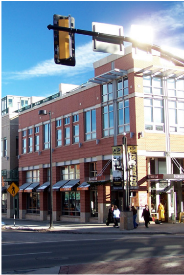
A parking garage in Denver, Colorado that blends in well with its surroundings. The parking garage also contains retail space.
