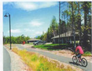
Figure 5: Swale in the Ty-Histanis Neighbourhood Development. The vegetated swales "infiltrate and convey stormwater and enhance safety for pedestrians/cyclists" (Canadian Mortgage and Housing Corporation, 2013, p. 4).
