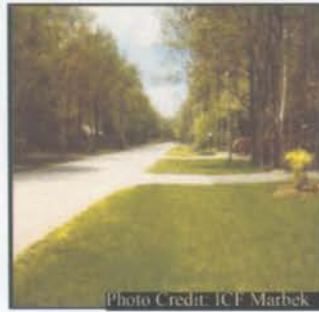
Figure 6: Grass Swale and Perforated Pipe Drainage in Ottawa (20 years).
