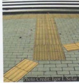
Figure #6: Changing direction or proceeding towards the intersection. The continuous dotted yellow line at the edge indicates a complete stop before crossing
