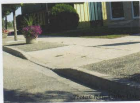
Figure #2: Return curb located outside the pedestrian walkway
