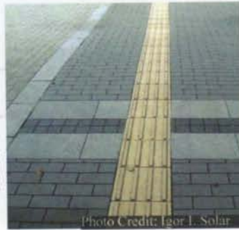
Figure #5: Tactile Ground Surface Indicators. No obstacle, just proceed straight ahead
