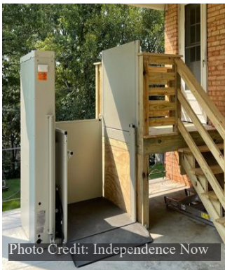
Figure 7: Automatic porch lift next to a stairway leading to an elevated door
