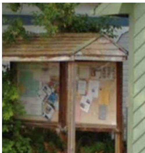
Figure 5-33. Right.. The current condition of the Rossburn billboard.
