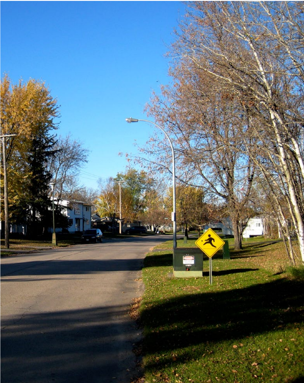
Identified safety concerns on path/street intersections
