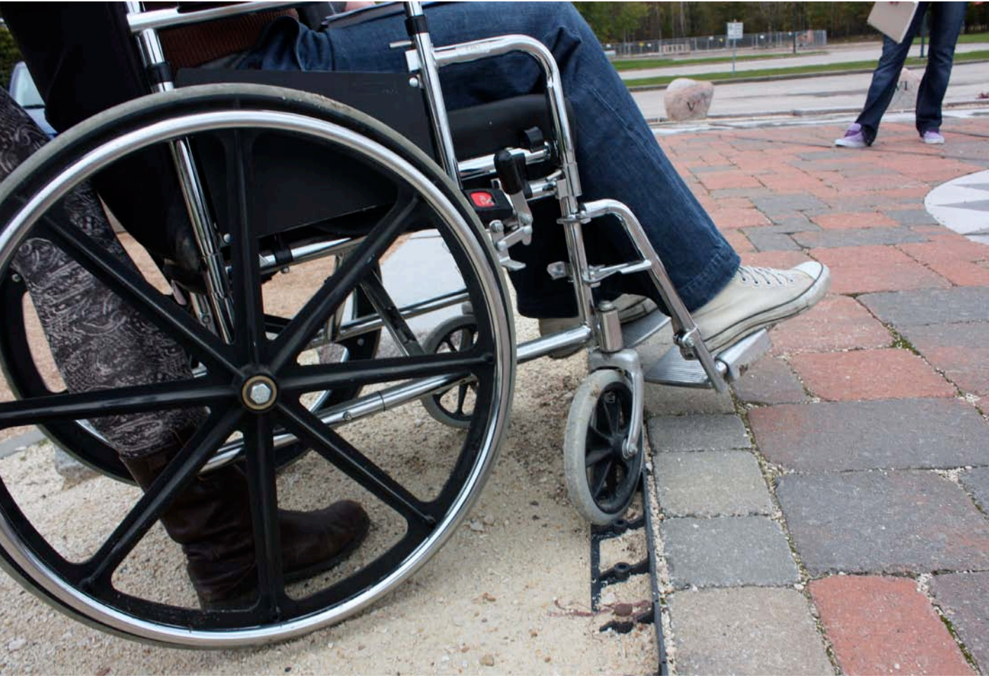
Irregular Trail/Road Intersection, Pinawa, MB
