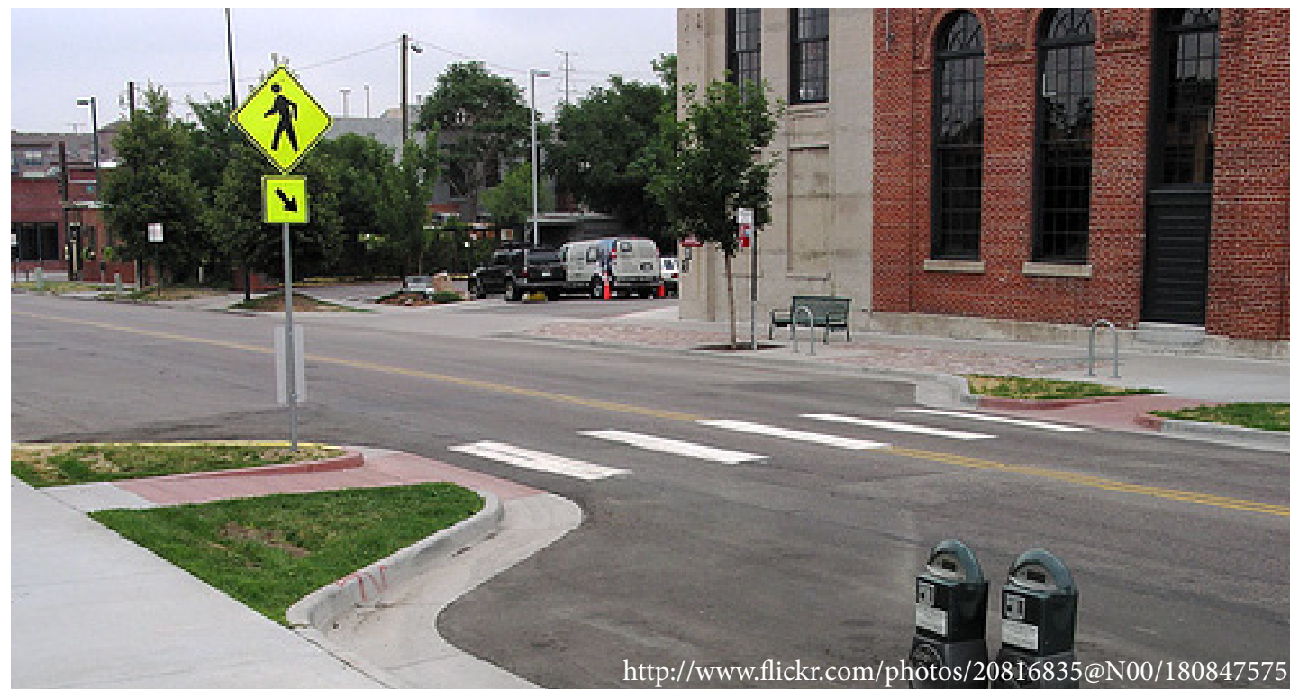
Bump outs slow traffic by narrowing the street, shorter street crossing
