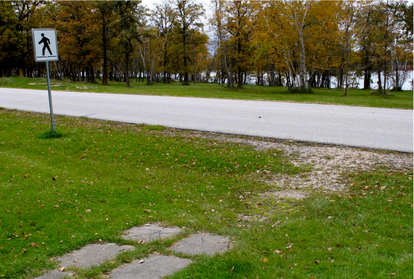
Irregular Trail/Road Intersection, Pinawa, MB
