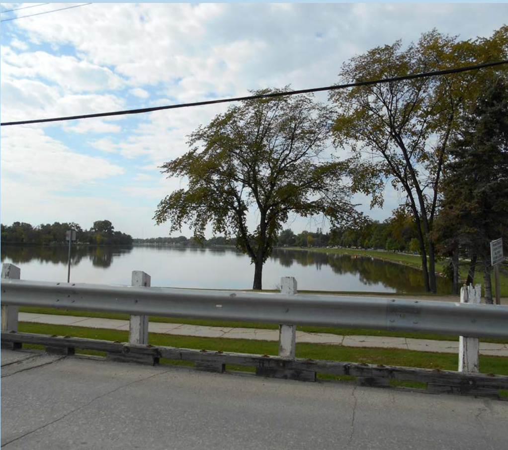
Island Park Bridge
