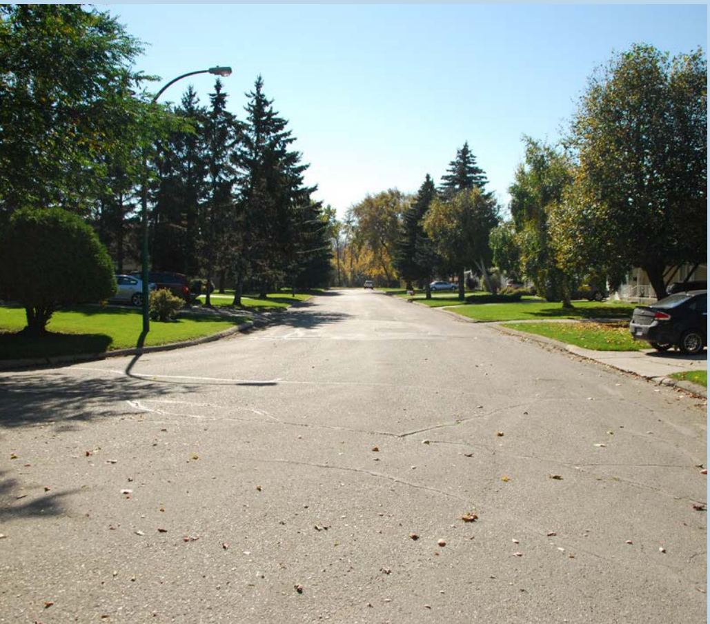
Residential road lacking sidewalks
