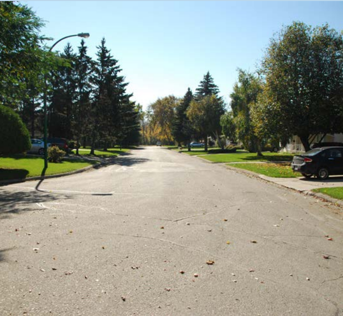
Residential road lacking sidewalks
