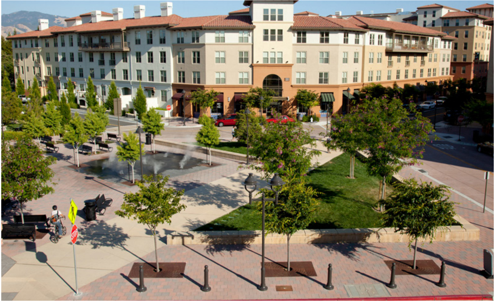
Transit Village Town Square, Contra Costa, CA.
