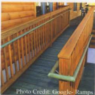
Figure #1: Zero-threshold concept with handrails
