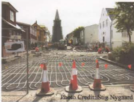
Figure 7: A snowmelt system being installed in Reykjavik, Iceland.
