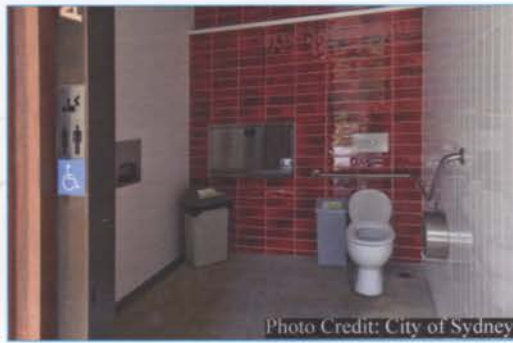
Figure 3: Public toilet illustrating inclusive access, large internal circulation space, and inclusive fittings and fixtures.
