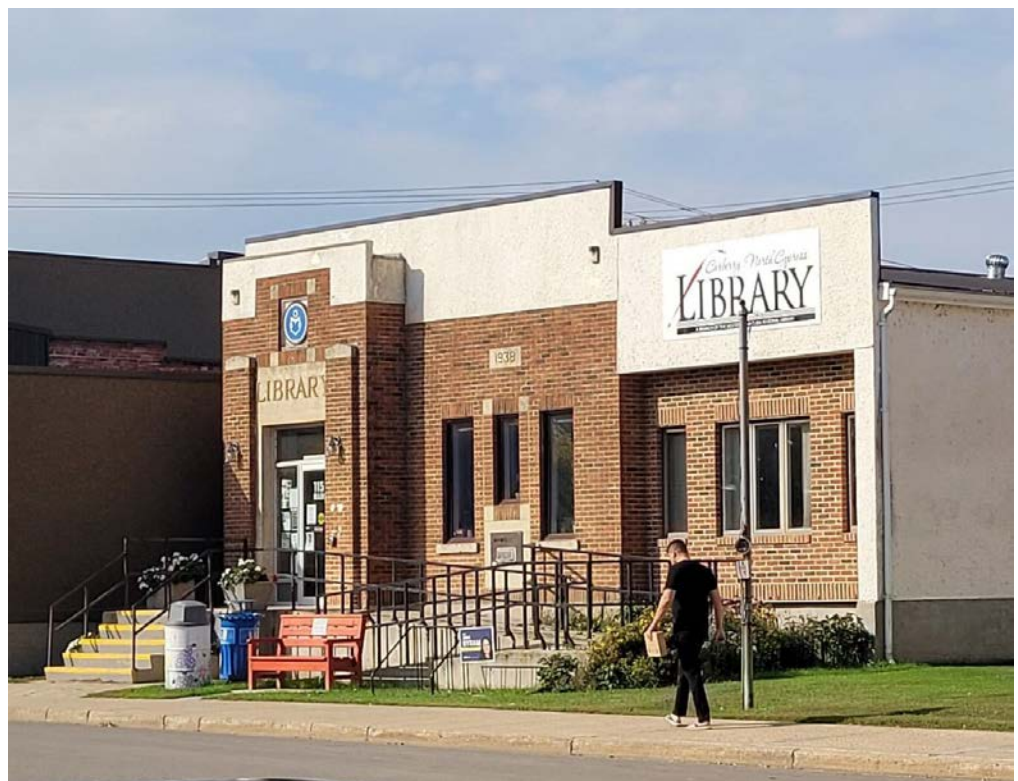
Figure: 15. Accessible ramps can be found on many buildings through town, including the library.
